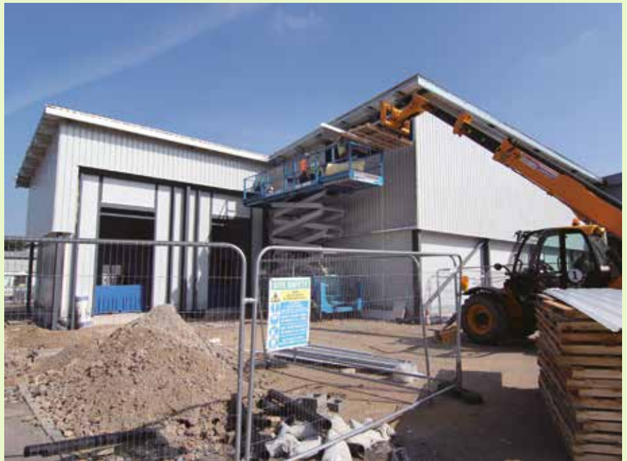
Building extension in Northampton, September 2014
