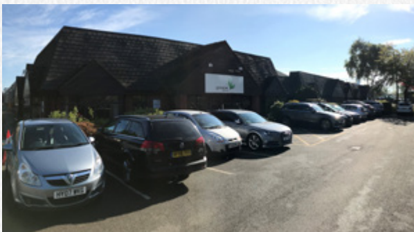
Our Greencore site in Spalding
